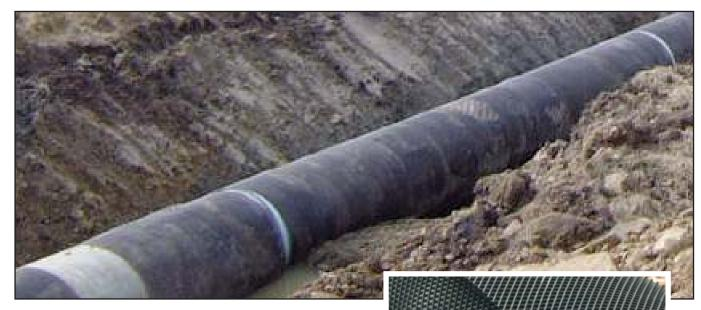
Denso Rockmesh is an expanded high density polyethylene mesh designed to give extra mechanical protection to pipe coatings laid in rough/rocky ground or abrasive backfill. Its diagonal mesh construction gives great flexibility for easy application whilst ensuring maximum protection to the pipe coating.
