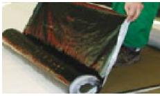
5. Torch lay the slate coated polymer-bitumen membrane facing upwards on Autotene Base
